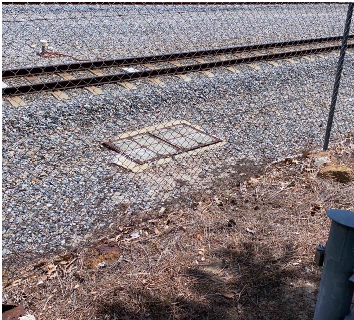
Telstra Manhole inside rail corridor (within 1m of active tracks) requiring special permits and closing the tracks for hauling
