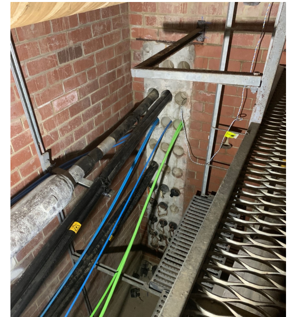
Super deep manhole, special works required to work in it
