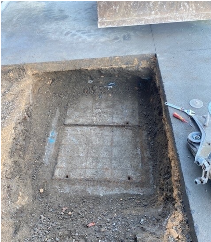
Telstra manhole concreted over by property developer
