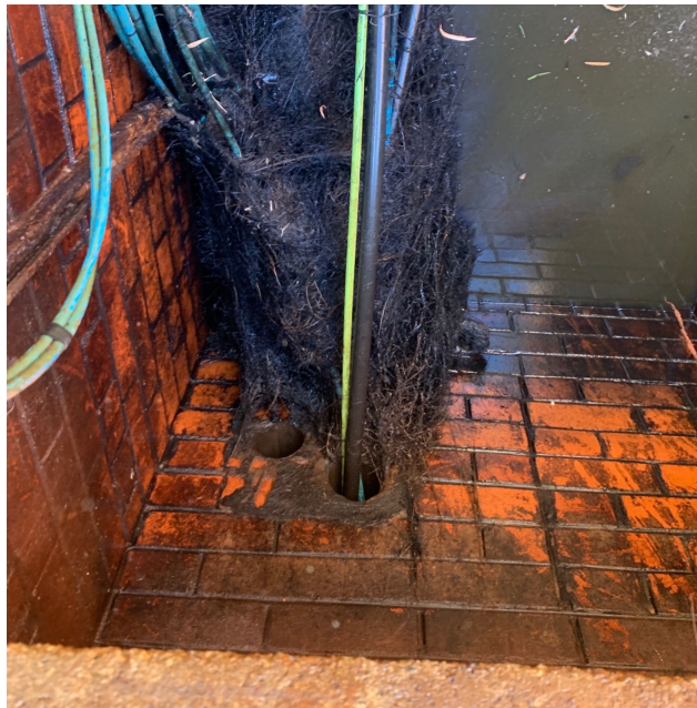
Tree roots inside Telstra manhole
