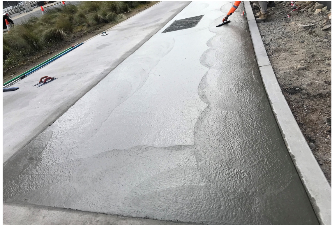
Aussie needed access to the manhole, so we lifted and aligned it with the new footpath and re-concreted the area.
